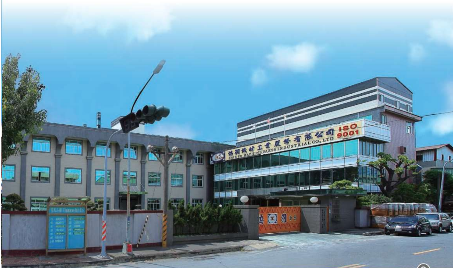
Kaohsiung Plant II
