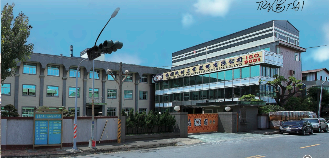
協羽高雄二廠 Kaohsiung Plant II
